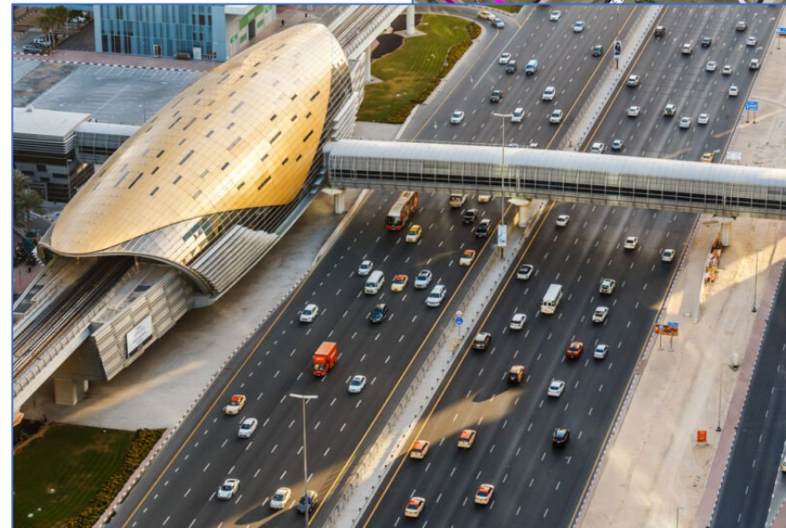
Dubai Mall Elevated Footbridge from Burj Khalifa Metro Station
