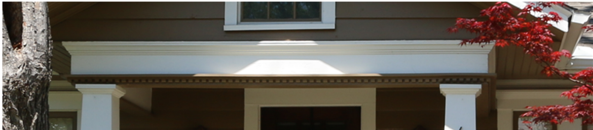
Examples: Minimum 8-inch header beam.
