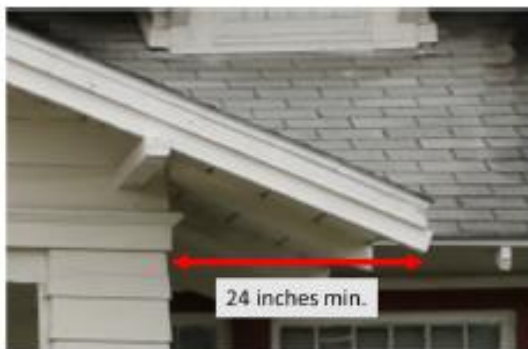
Example: Roof eave must be a minimum of 24 inches.
