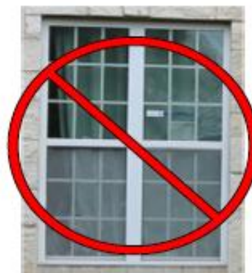
Example: Window grilles behind the glass are not typical of the Craftsman style.
