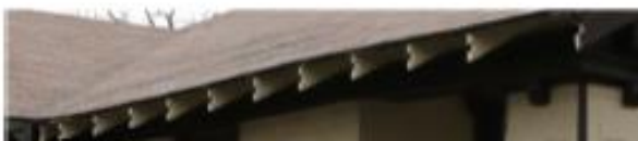
Example: Roof eave must be a minimum of 24 inches.
