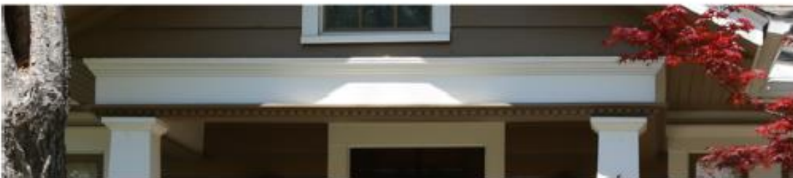
Examples: Minimum 8-inch header beam.
