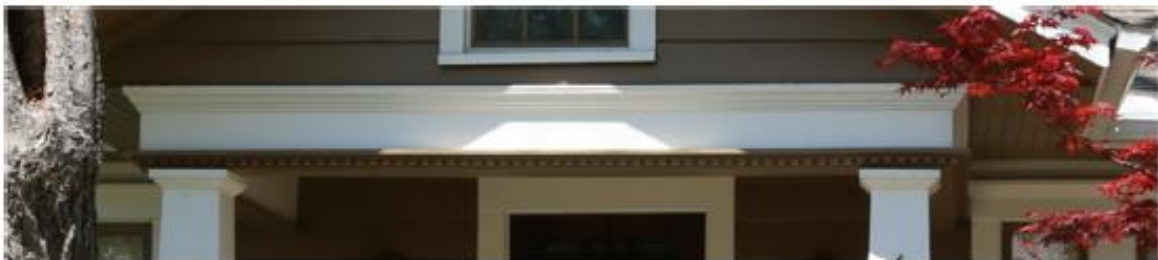
Examples: Minimum 8-inch header beam.
