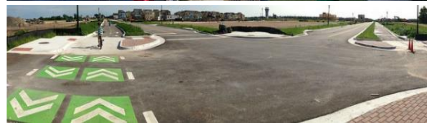
Protected intersection with separate bike lanes
