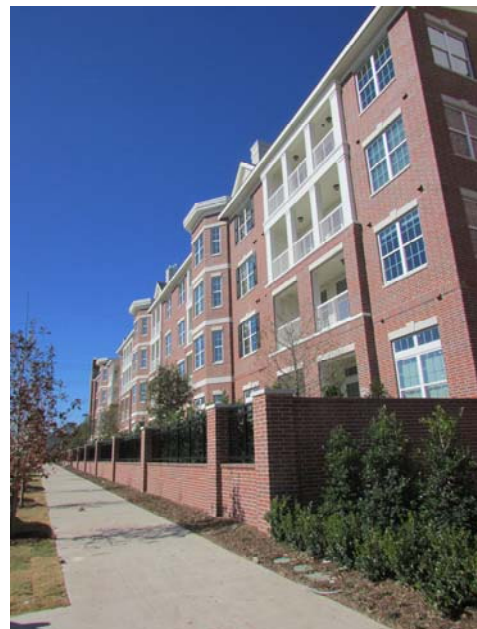
Traditions senior living (right), part of the Signature Pointe redevelopment in the Mockingbird Sub-District
