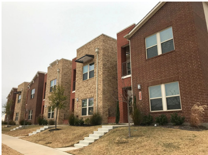
Fiji Townhomes completed in 2017.
