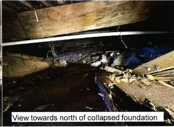
NE Workroom Floor Damages
