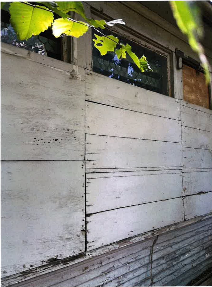
Figure 22 - Partial view of the north side projecting bay showing evidence of fenestration patterns and character (photograph taken July 25, 2022)
