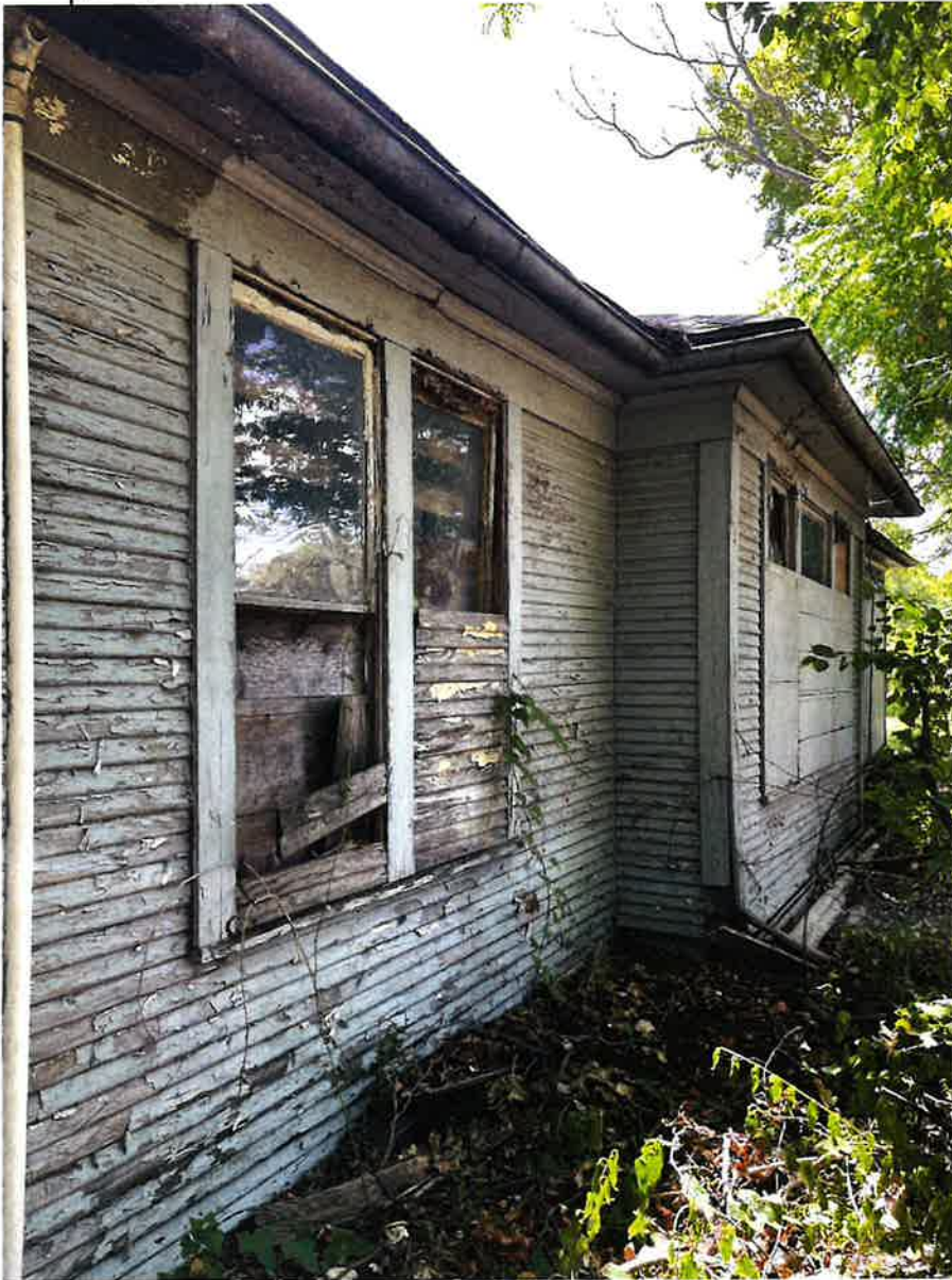
Figure 7 – Partial view of the north elevation (photograph taken July 25, 2022)
