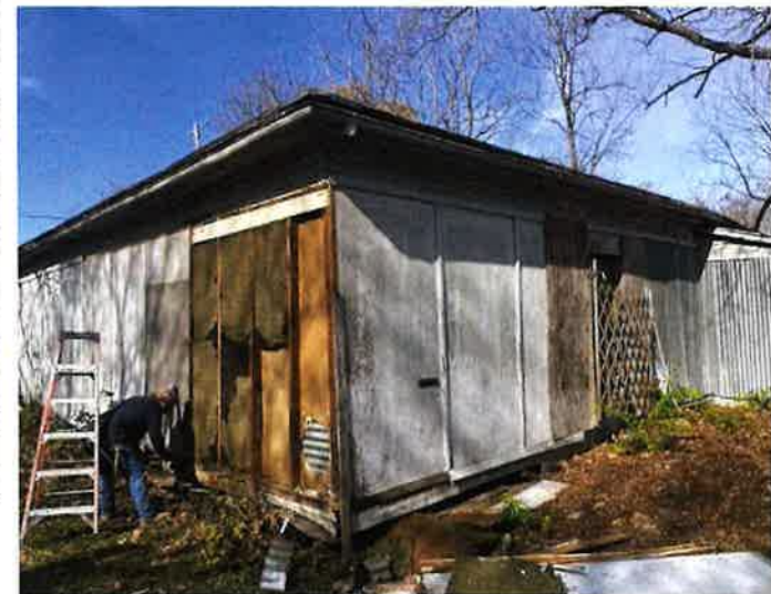
Exposed bay shows no evidence of balustrade or columns
