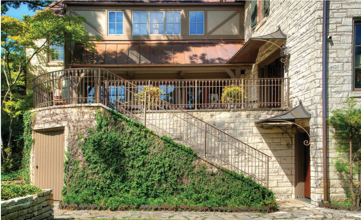
Figure 12: Detail of three-story east elevation with terrace. July 2021. Photography by Carolyn Brown.
