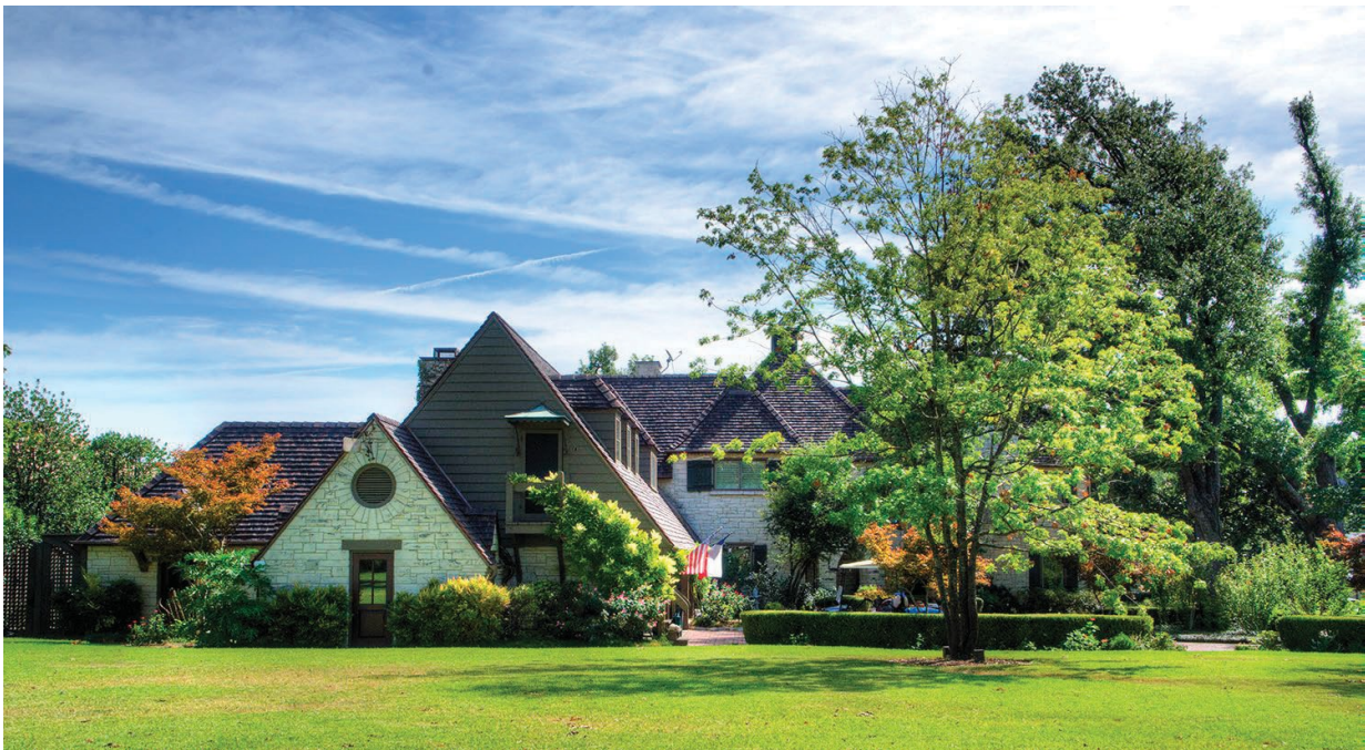
Figure 2: West elevation, facing Strait Lane. July 2021. Photography by Carolyn Brown.
