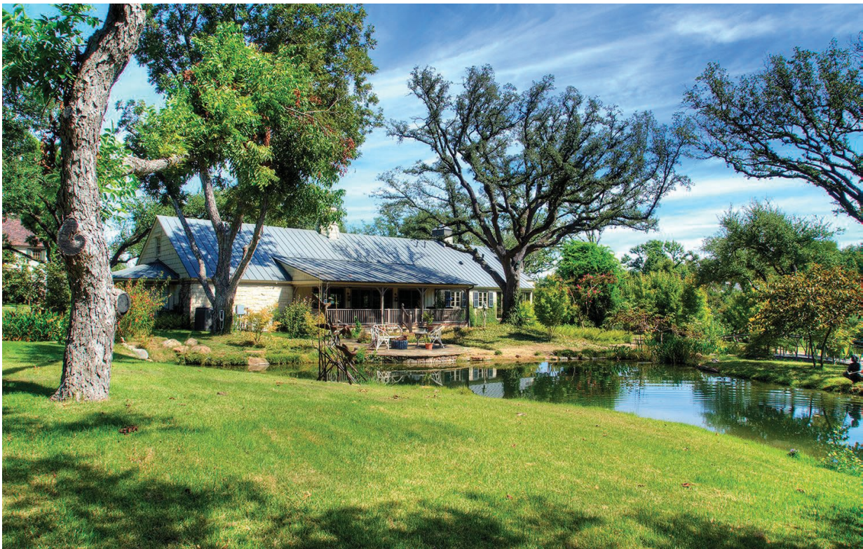
Figure 19: Non-historic accessory structure used as party barn. July 2021. Photography by Carolyn Brown.
