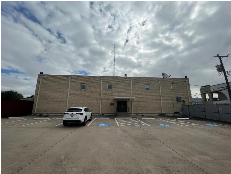
Exterior from back of building that will be new main entrance
