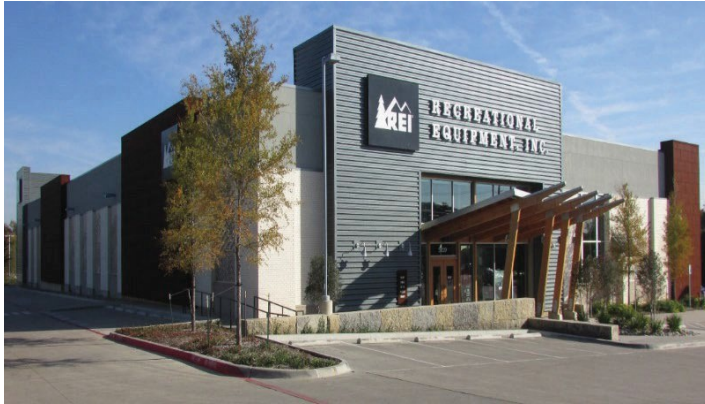
The REI sporting goods store that was built as part of Half Price Books’ multi-phase plan to redevelop the former Parker Plaza site
