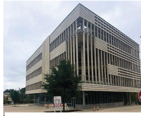
Construction of BookMark Center retail and office space as part of Half Price Books’ multi-phased development is complete and available for lease.
