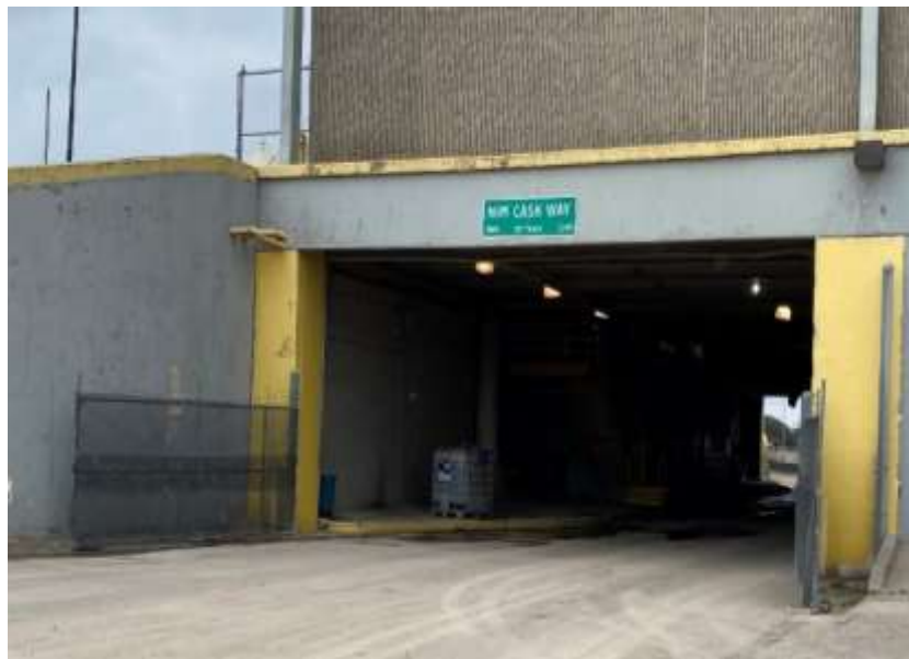
Figure C-8: Transfer Trailer Tunnel at Bachman Facility
