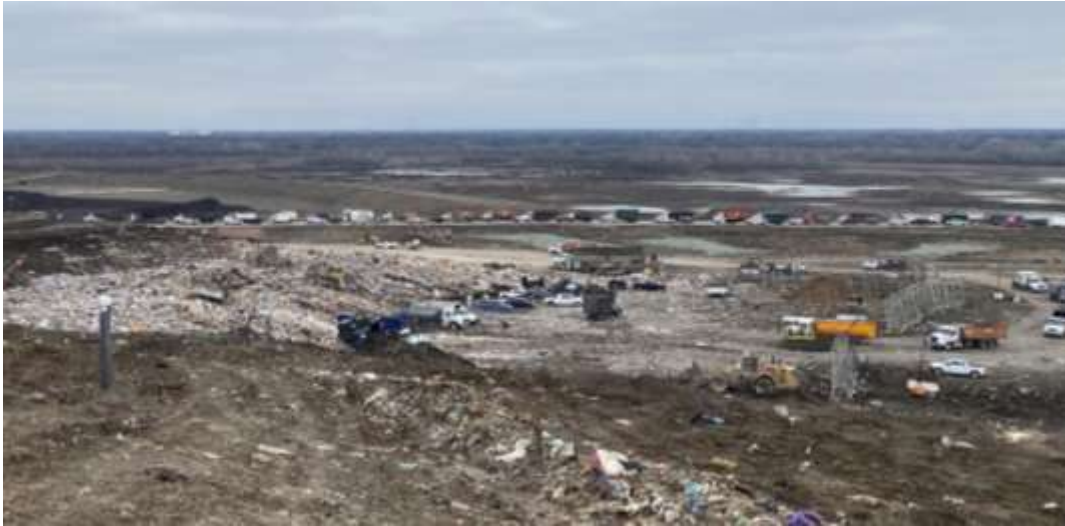
Figure E-14: Landfill Working Face and Vehicle Queue
