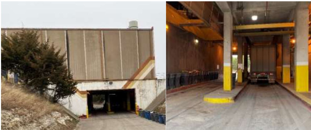
Figure C-19: Westmoreland Facility Transfer Trailer Truck Pull Through Location
