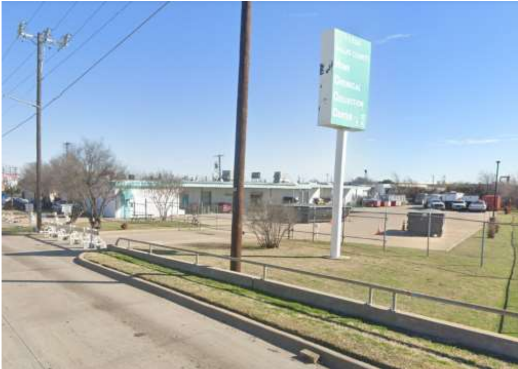
Figure 12-1: Dallas County HCCC
