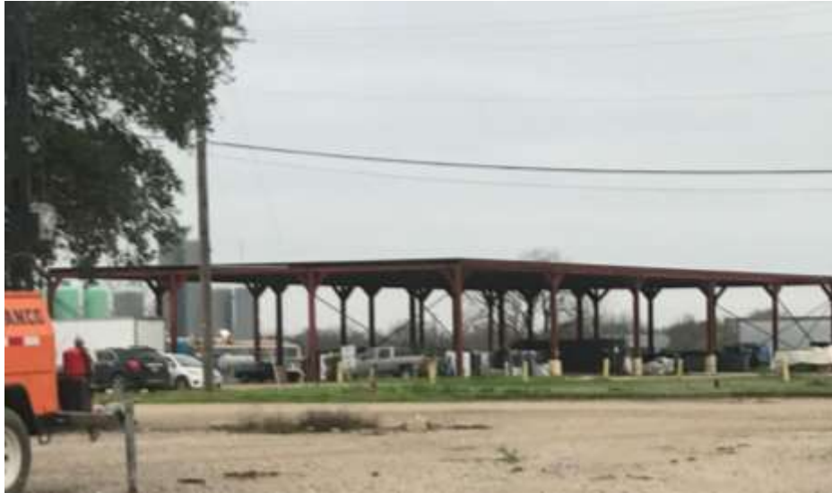
Figure E-20: CCRC Permanent Pole-Barn Structure
