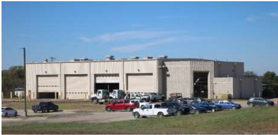
Figure E-3: Heavy Equipment Maintenance Shop
