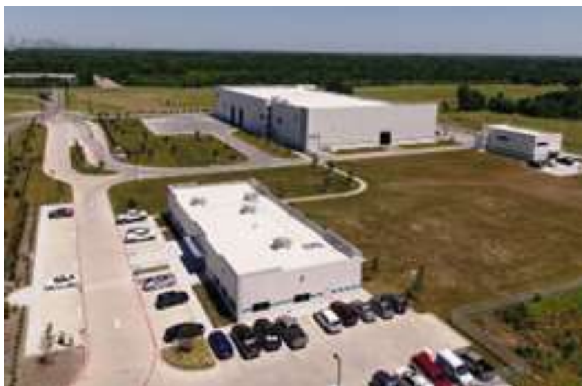
Figure 4-4: MRF Building Located at the Landfill
