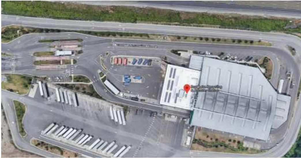
Figure 5-2: Bow Lake Recycling & Transfer Station
