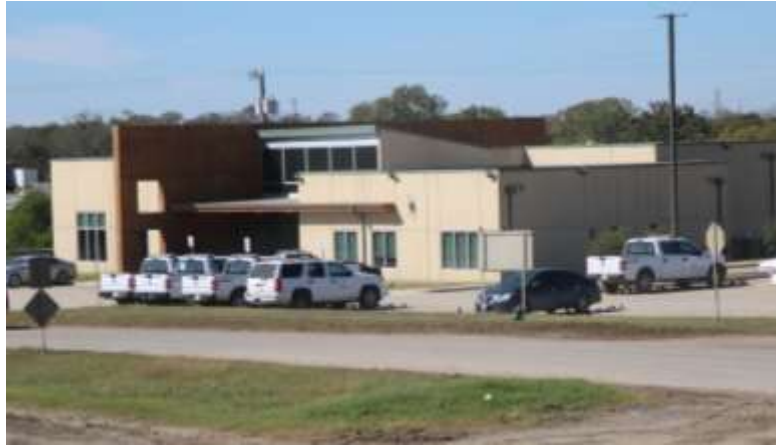
Figure E-22: Administration Building
