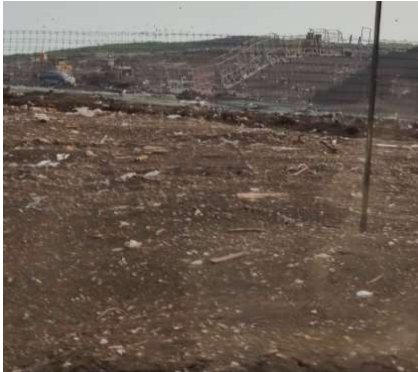
Figure E-24: Mobile Litter Control and Secondary Litter Control Fences
