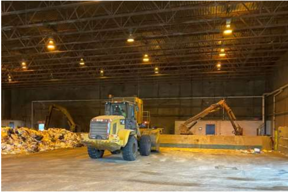
Figure C-18: Westmoreland Facility Hoppers
