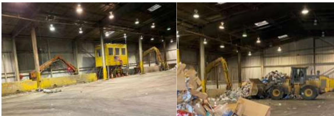
Figure C-13: Fair Oaks Facility Tipping Area
