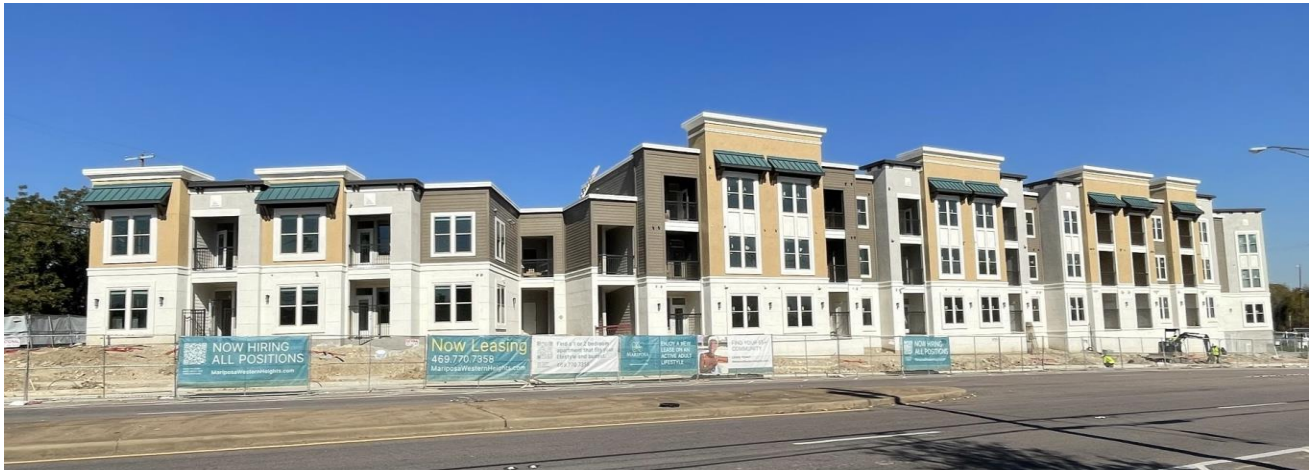
Mariposa (Villas) at Western Heights (under construction)
