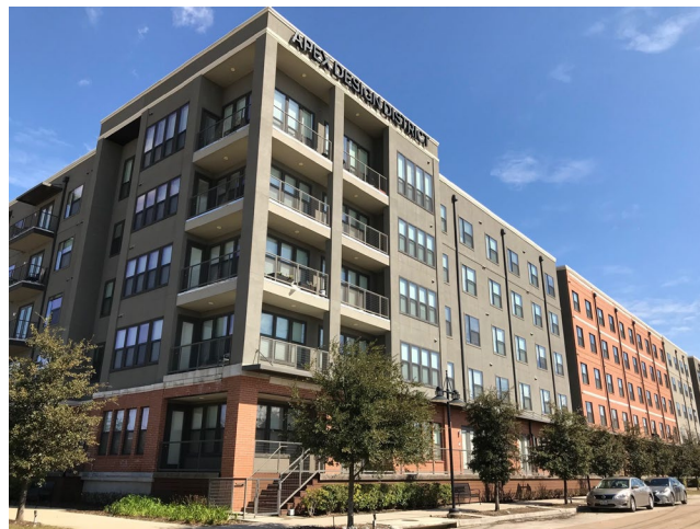
Alexan Riveredge (now Factory Design District) at 120 Turtle Creek Blvd.
