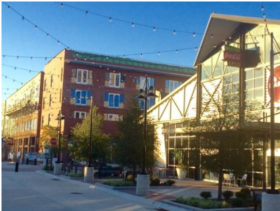
Street view between Taylor Building and Farmers Market Shed 2 Harvest Lofts (Shed 3 and 4) in distance
