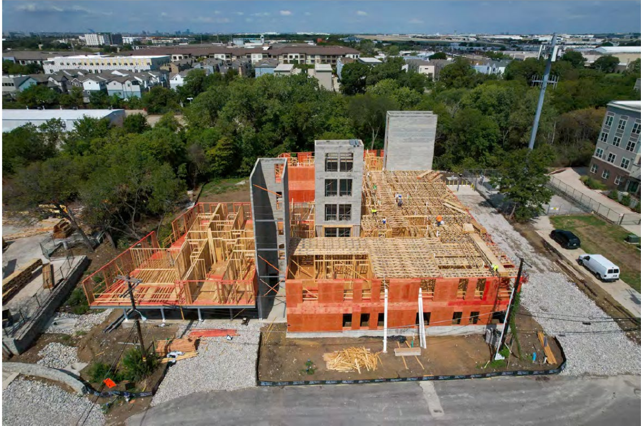
Oak Lawn Place – Under Construction
