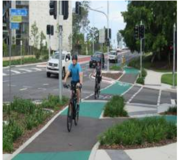
Raised bike lanes protect cyclists and provide an easy path of travel.
