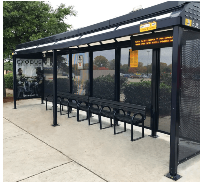
Covered bus stops with benches provide comfort to users.
