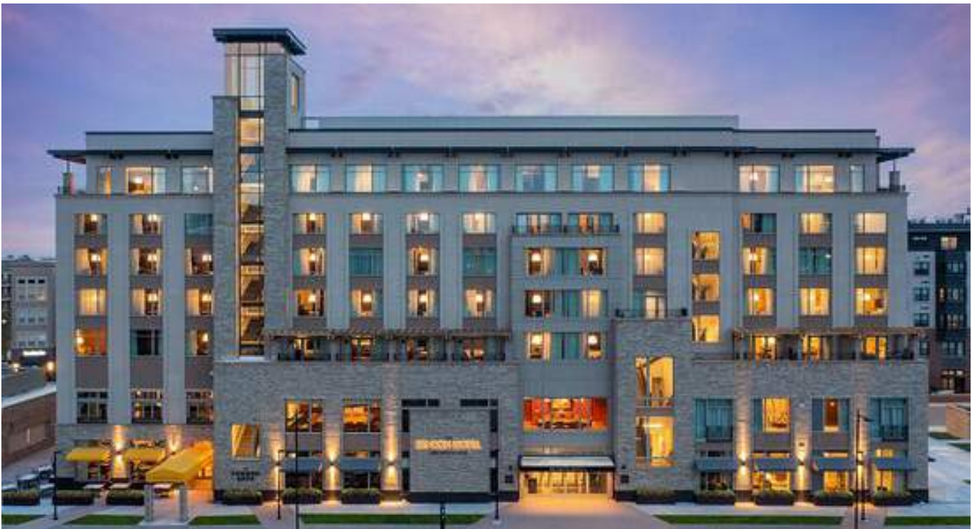
The hotel and event center will provide views overlooking the Town Center.
