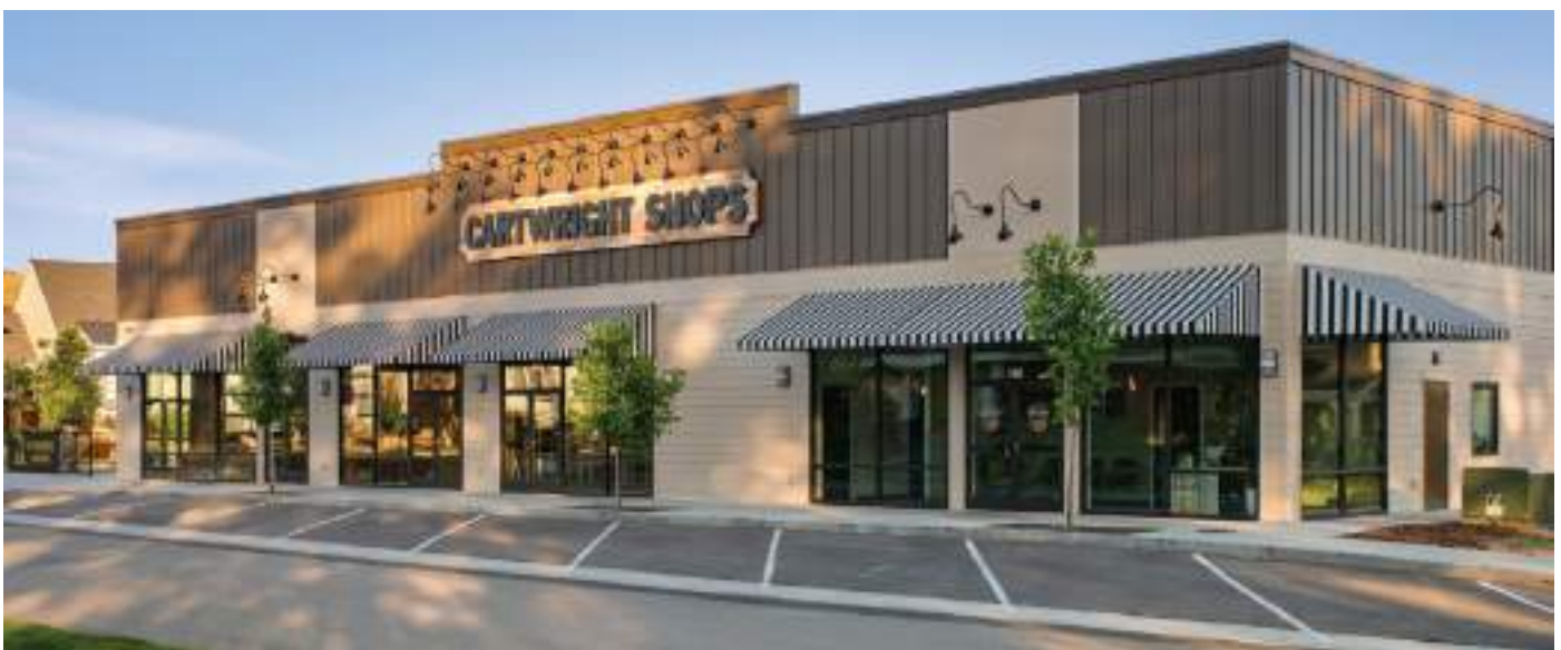
Strip retail buildings
