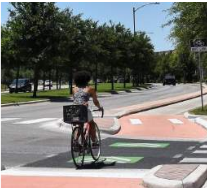
Raised Bike Lanes in Austin, TX foster a safe environment for cyclists, reducing conflicts with vehicles and pedestrians.
