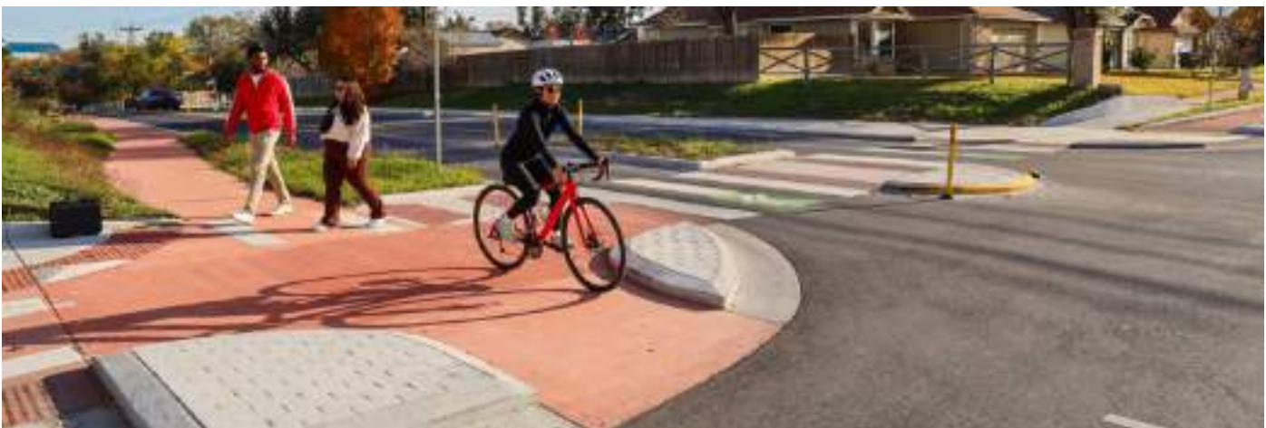
Raised bike lanes help protect cyclists, motorists, and pedestrians.
