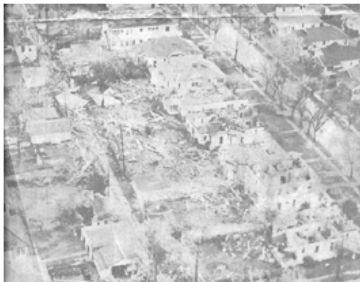
The 1957 Oak Cliff tornado damaged numerous homes in the West Oak Cliff Area
