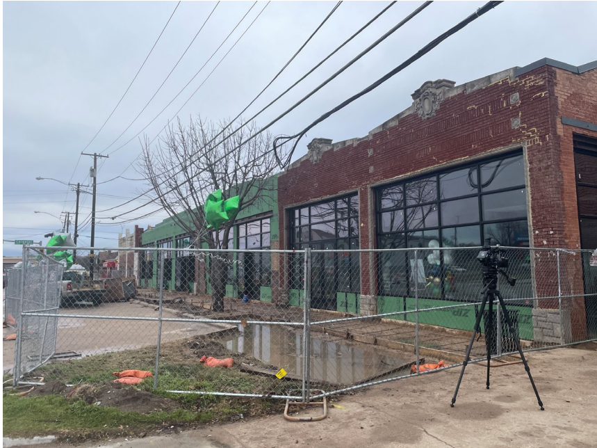
Retail building renovation at 1632 Martin Luther King Jr Boulevard.
