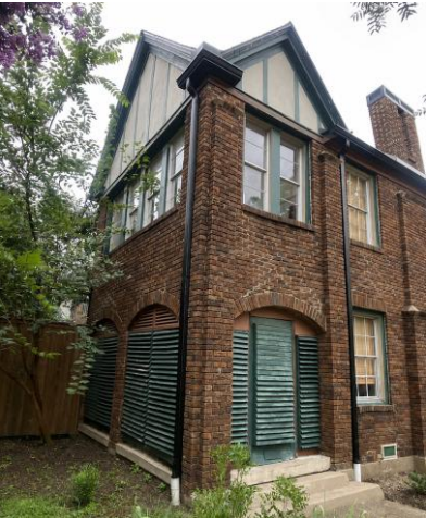
Current louvers and screens, view facing Junius St
