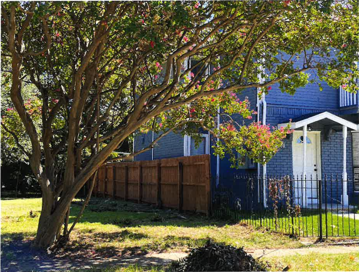
Close up of right (northeast) side of subject property.
