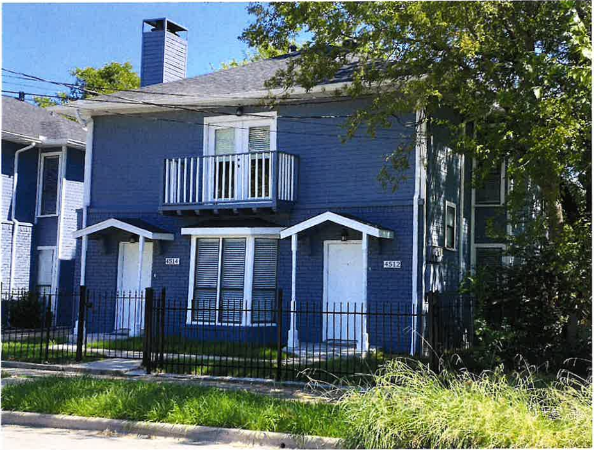
Close up of left (southwest) side of subject property.
