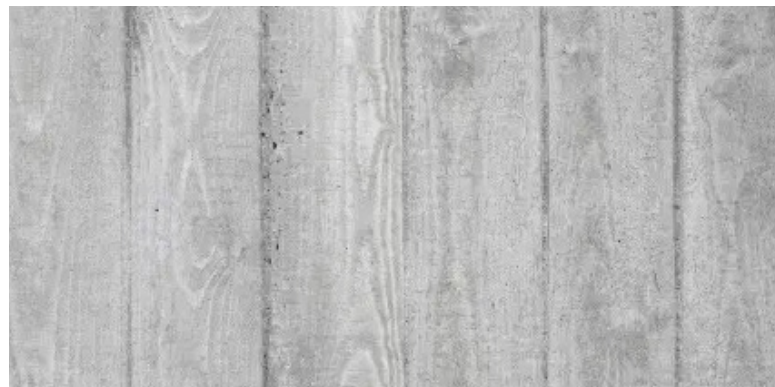
Concrete 1 Vertical board formed
