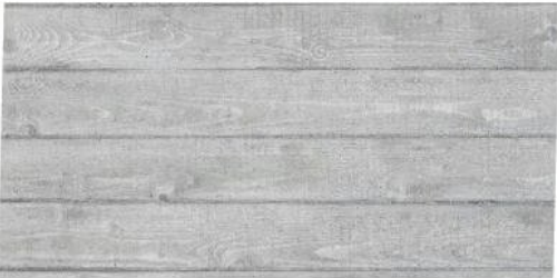
Concrete 1 Horizontal board formed
