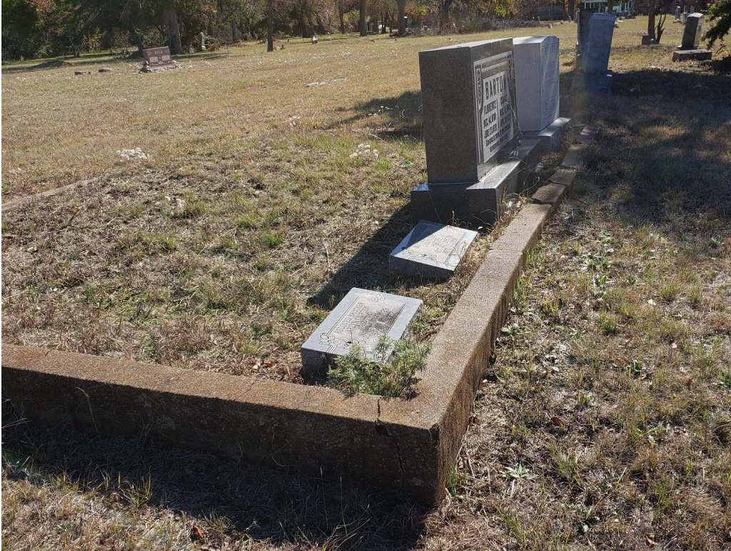
Photo 10. Example of a Concrete Curb Plot (Barton Family). Courtesy of Sheniqua Cummings, Nov. 18, 2019.
