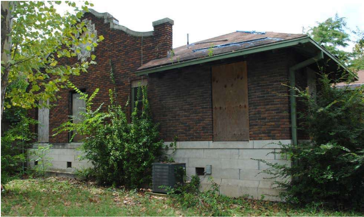
Figure 6. Bianchi House, Northeast Elevation, August 2017
