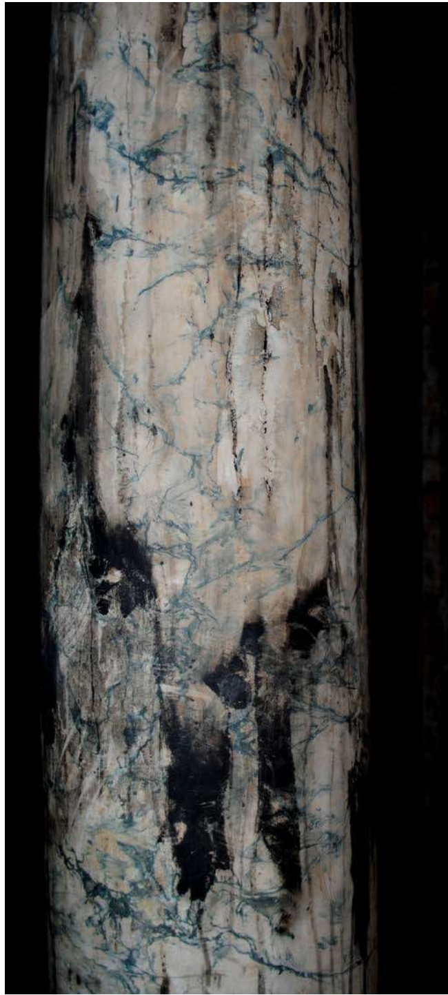
Figure 13. Close-up of Scagliola Column
