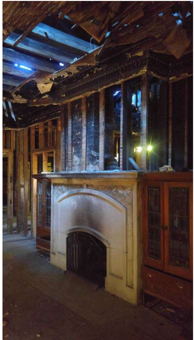
Figure 11. Fireplace and Mantel (Photos: Norman Alston, ALA)
