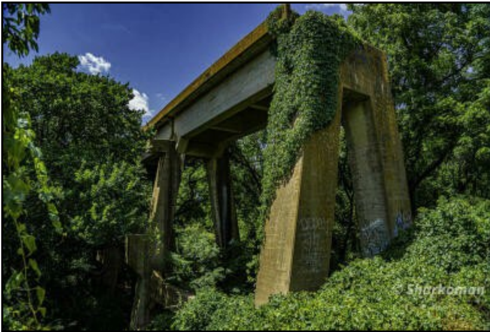
Figure 3. Photo showing the bridge substructure (courtesy of Jesse Sharkoman, June 2019, https://bridgehunter.com/tx/dallas/bh67825/ ).
