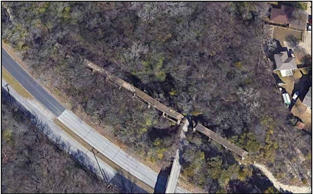
Figure 1. Aerial image of Mountain Creek Interurban Bridge (courtesy of Google Earth).
