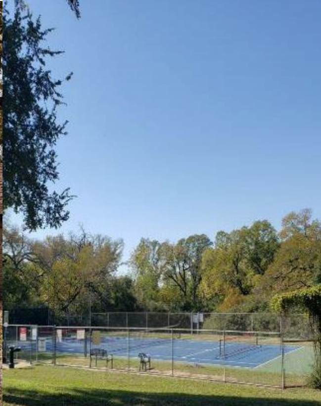
TENNIS COURT RESURFACING @ PENINSULA NEIGHBORHOOD (PMO)
