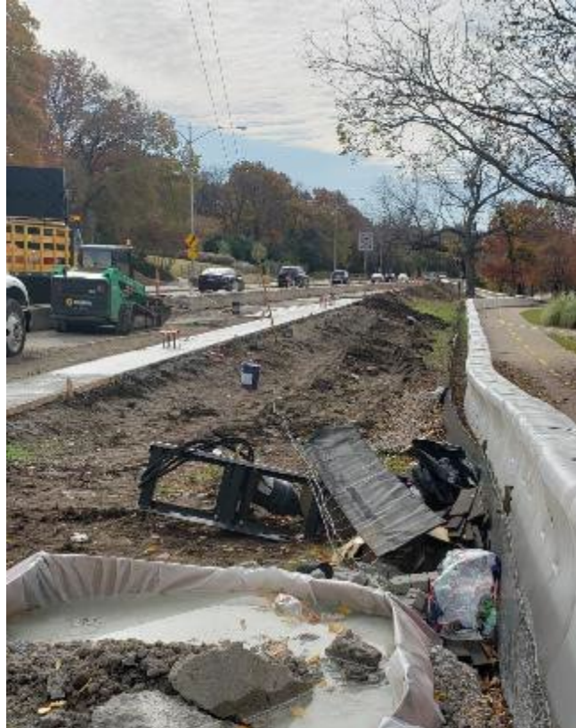
GARLAND ROAD TRAIL PROTECTION (FACILITIES, P&D, TxDOT)
