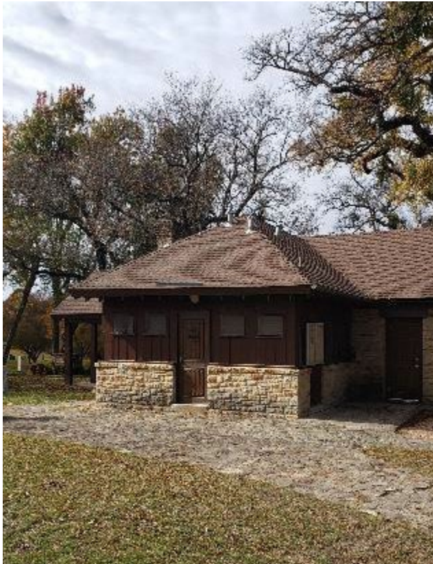
SUNSET INN RENOVATIONS (PMO AND FACILITIES)
