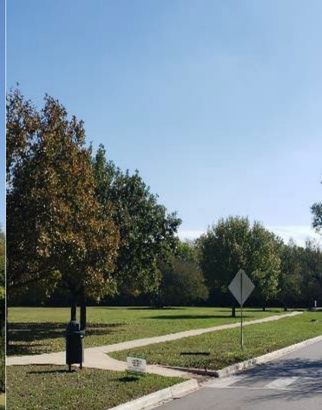
NEW PEDESTRIAN TRAIL @ WINSTEAD (PMO+PUBLIC WORKS)
