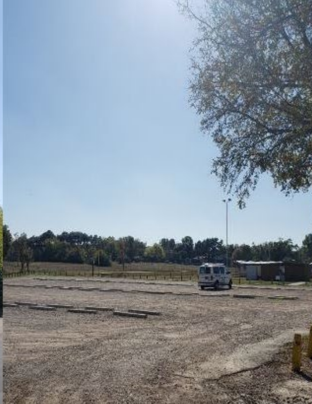
RENOVATED PARKING LOT @ WINFREY POINT BALLFIELD (PMO)
