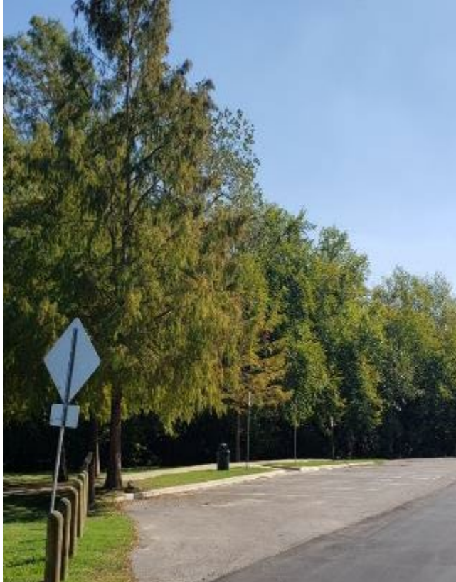
NEW PARKING LOT @ WINSTEAD (PMO+PUBLIC WORKS)
