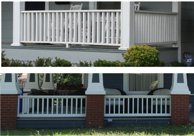
Examples: Wood balustrade on the front porch.
