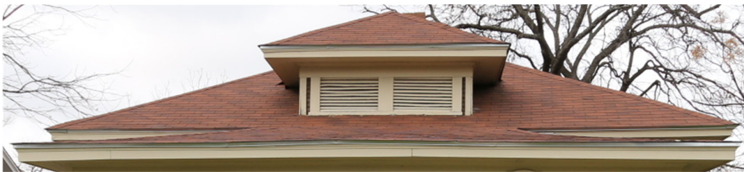
Examples: Centered, hipped dormer with louvered vent.
