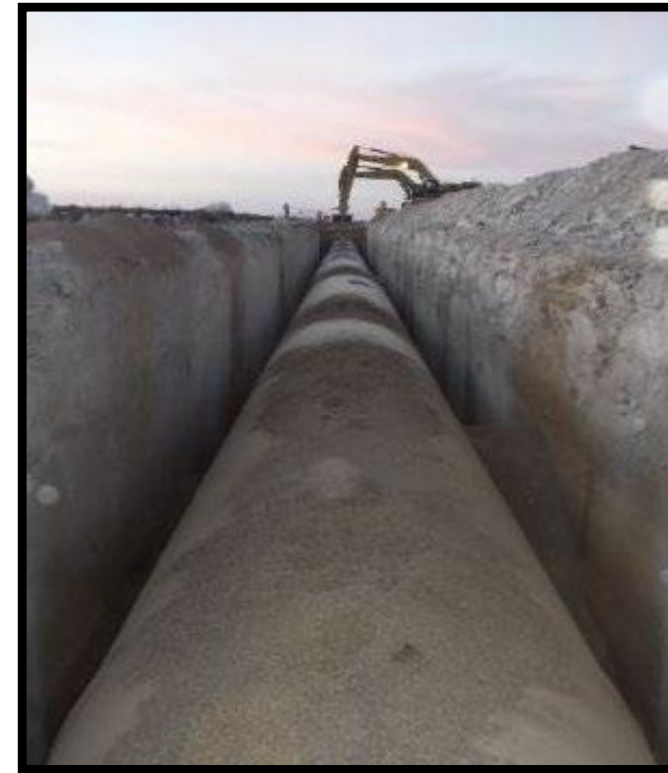
Installation of 108-inch pipe along IPL Section 17
