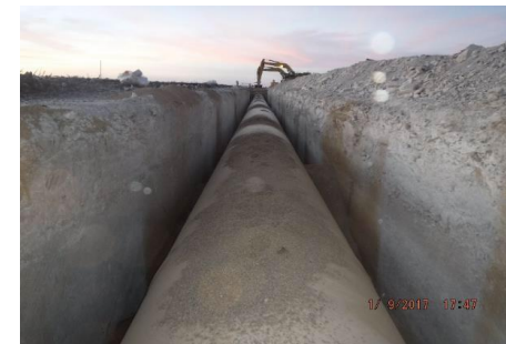
Installation of 108-inch pipe along Section 17
