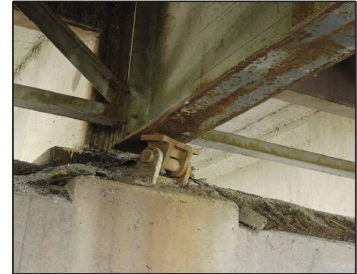
REFERENCE IMAGE AT TYPICAL MISALIGNED BEARING
