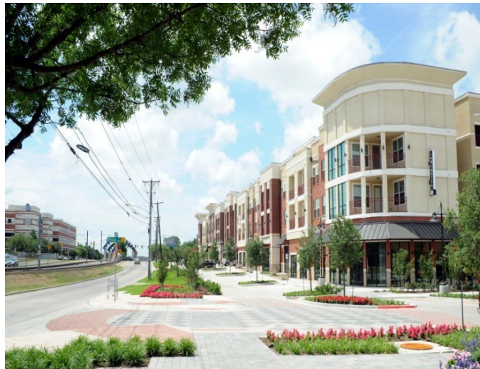
Lancaster Urban Village across from the VA Medical Center Station (southern Dallas)
