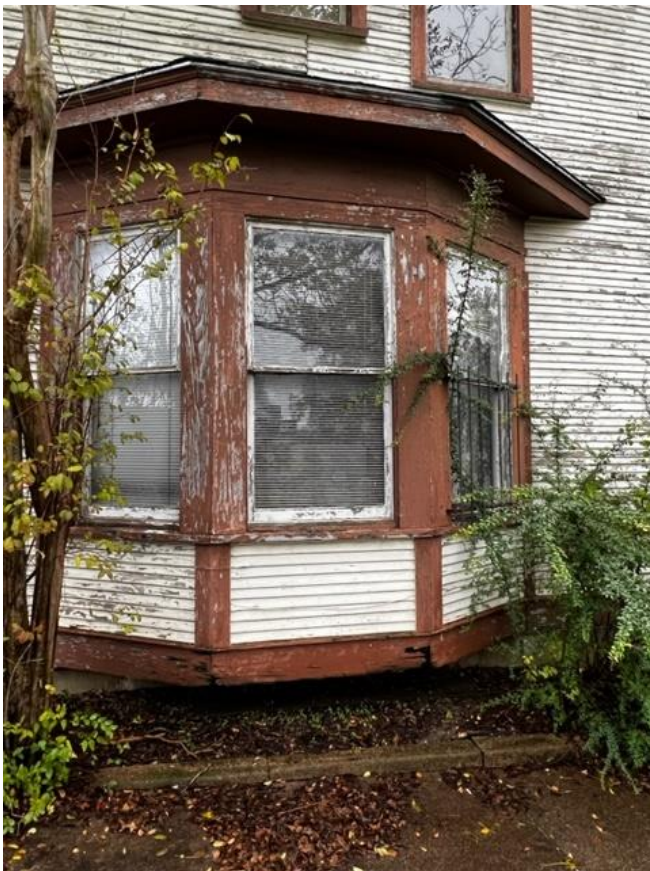
North Elevation – Failing Siding Visible
