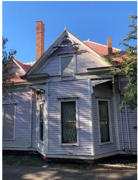
East Elevation (3 views) – Failed windows Damaged decorative detail visible
