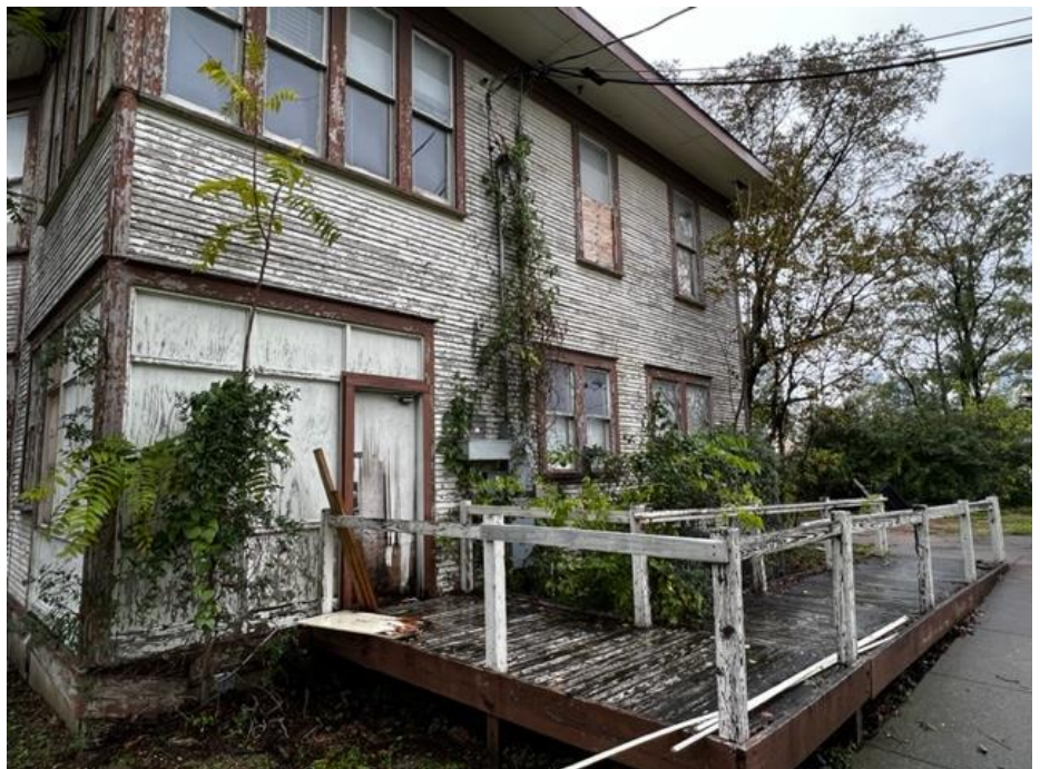
East Elevation (3 views) Failed Windows and Failed Siding
