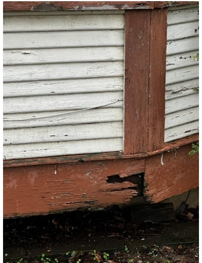
North Elevation – Failing Siding Visible
