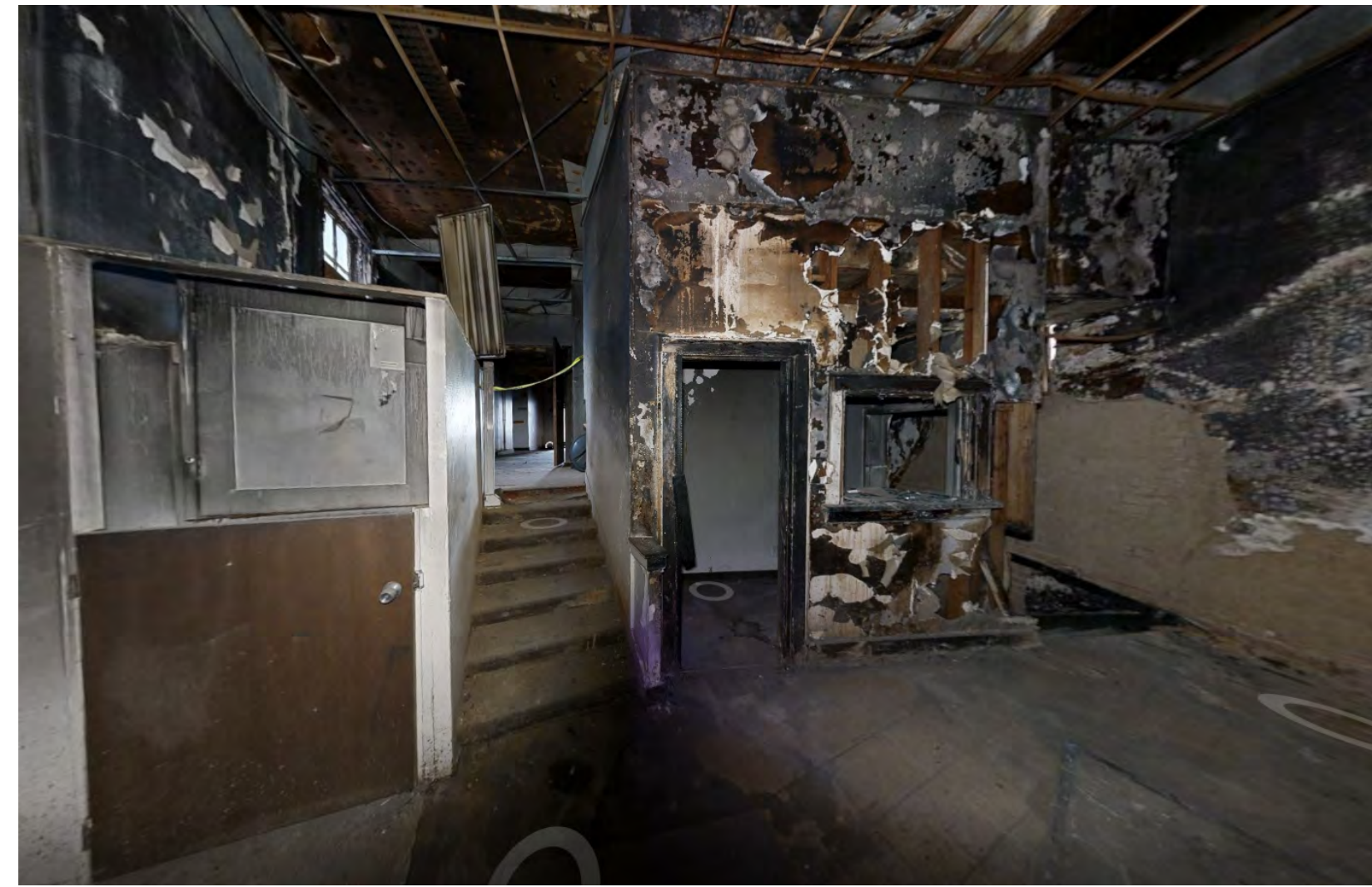
PHOTO_8 WHEELCHAIR LIFT
