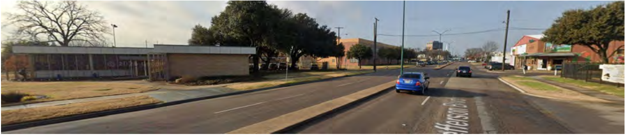
West of Oak Cliff UMC (subject property) along E. Jefferson Blvd. Source: Google Maps -- Streetview.
