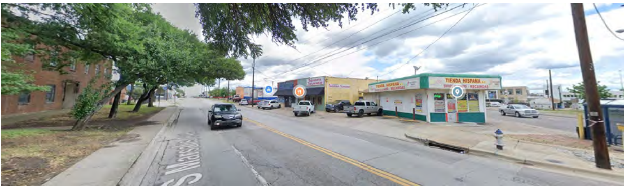
North of Oak Cliff UMC (subject property) along Marsalis St. Source: Google Maps -- Streetview.
