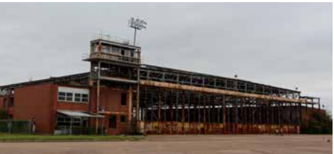
Dallas NAS Maintenance Hangar (1941)
