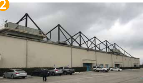
Aircraft Maintenance Hangar (1972-1979)
