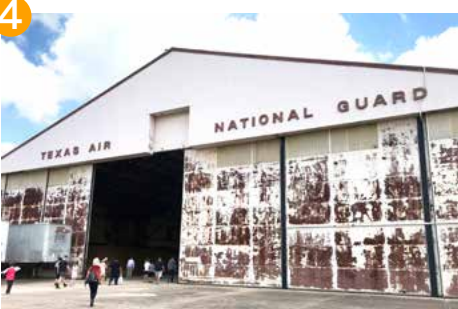
Texas Air National Guard Hangar (1961)
