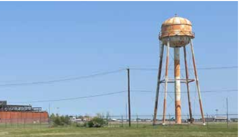
DNAS Water Tower (1941)
