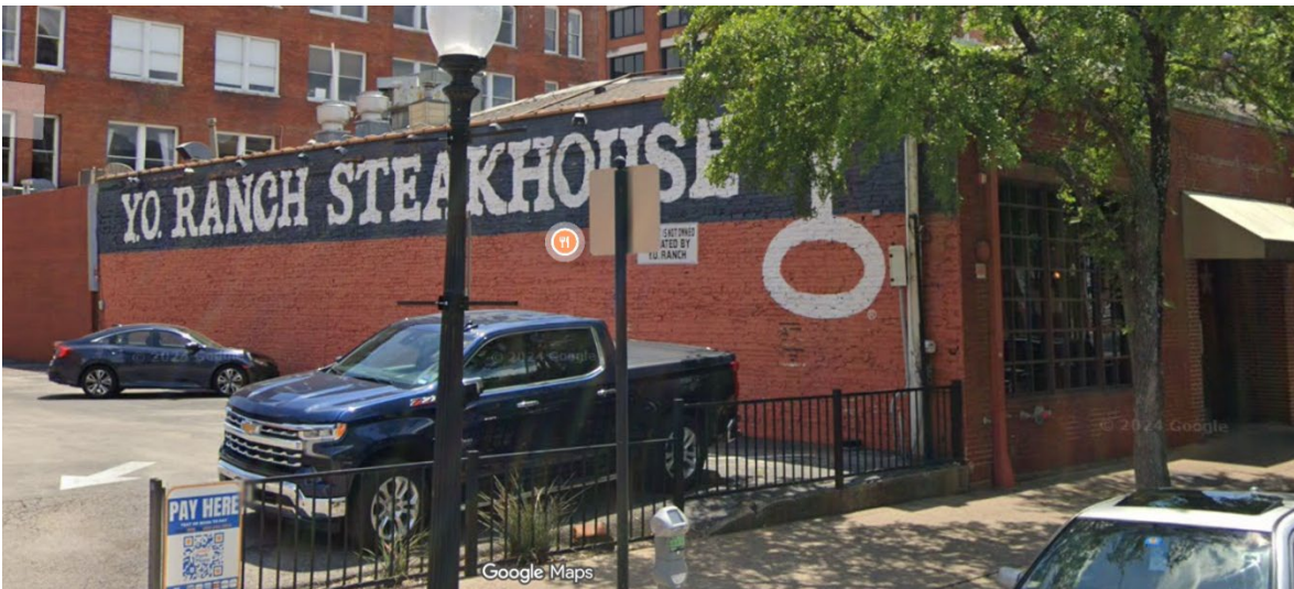
Subject property. East (left) elevation depicts a former shared/party wall. Source: Google Maps - Street View (Feb. 2025).
