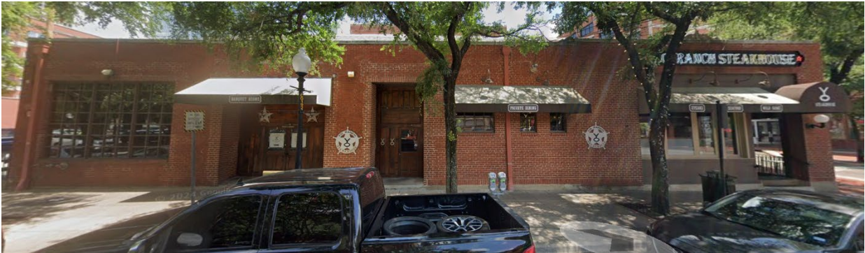
Subject property. North (front) elevation, Ross Avenue frontage (depicts storefront(s) and awnings). Source: Google Maps -- Street View (Feb. 2025).
