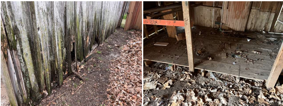
Pictures 1 - 6: General structural condition of detached structure.
