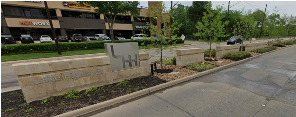
Skillman Street Median Improvements
