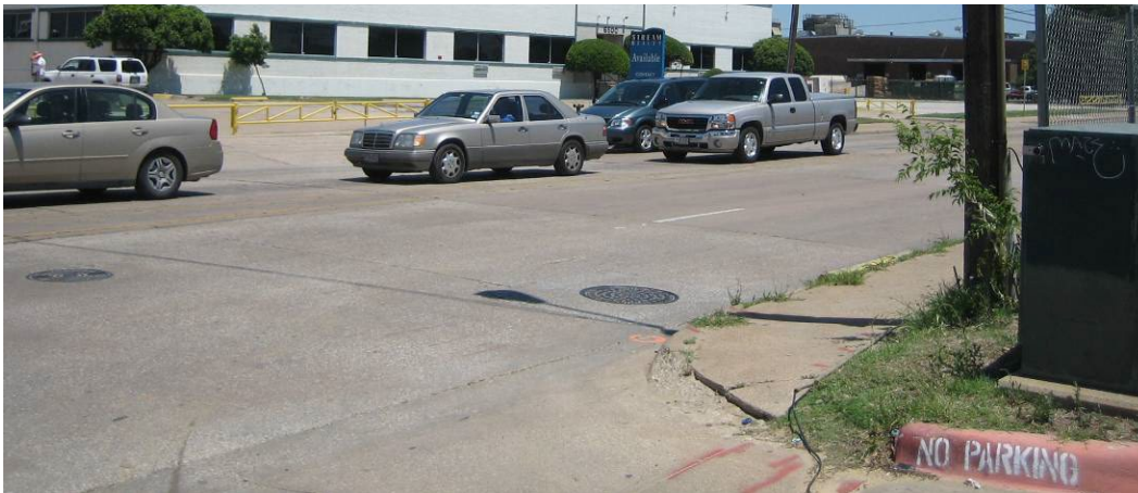
Crumbling curbs and a lack of pedestrian crossings
