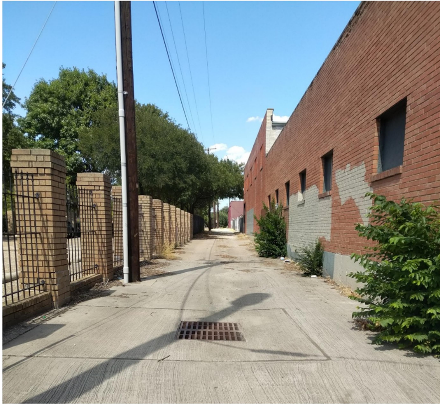
View of existing alley, looking north from Good Latimer Expressway
