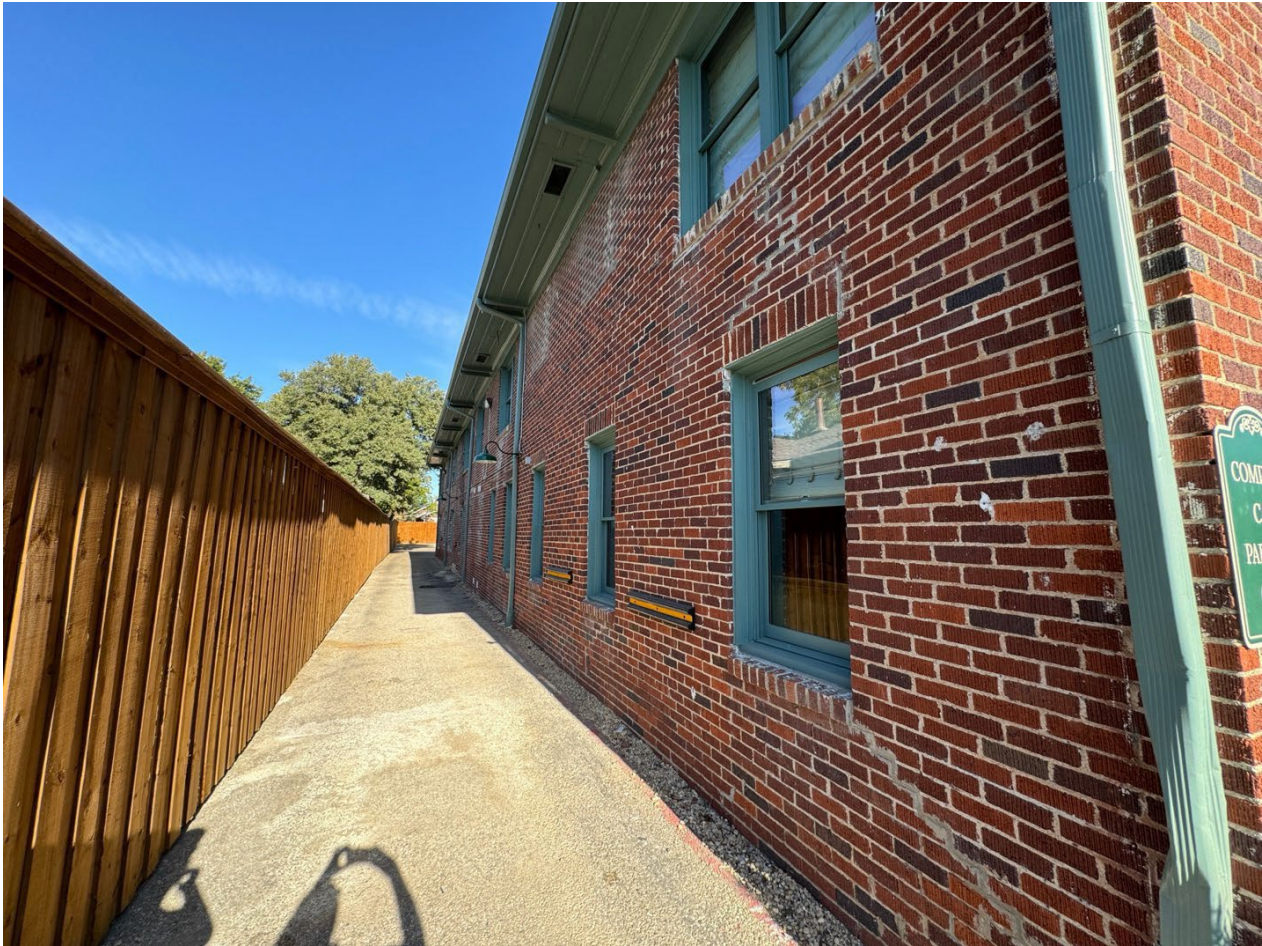
Image 3 - South elevation with drive facing west.
