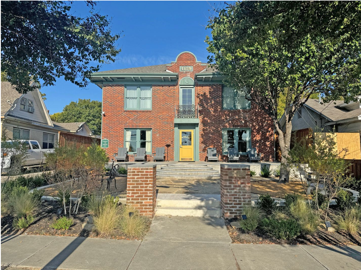
Image 2 - East elevation with yard and terrace
