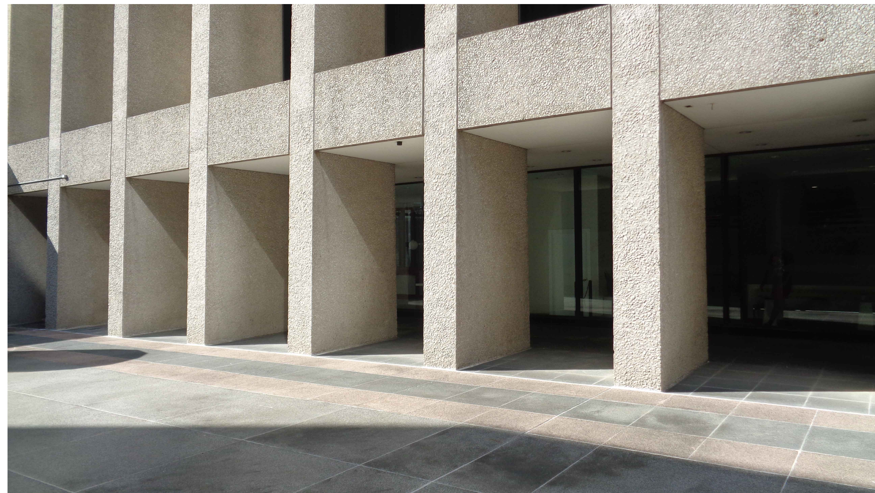
VIEW B - LOOKING WEST
