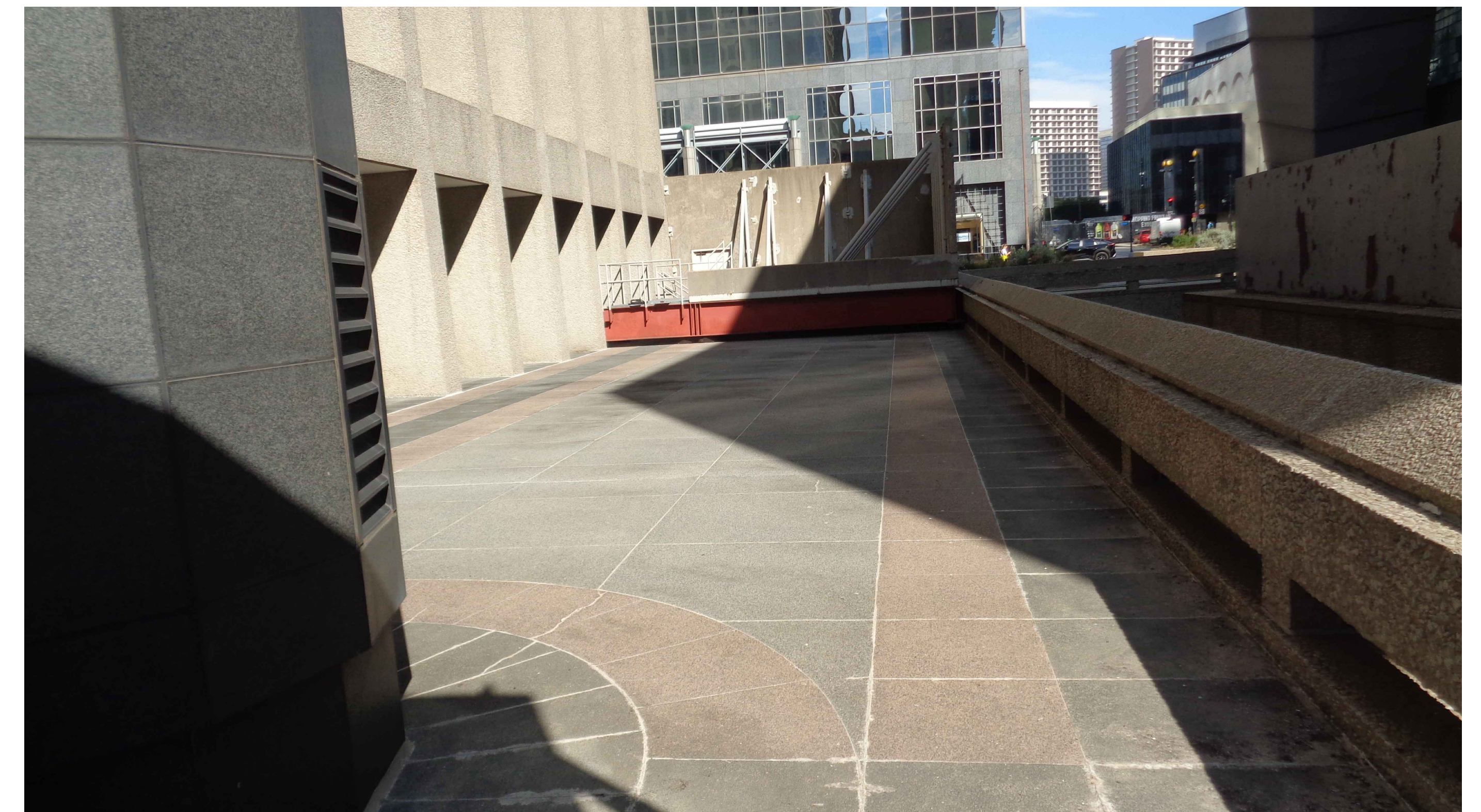
VIEW A - LOOKING NORTH
