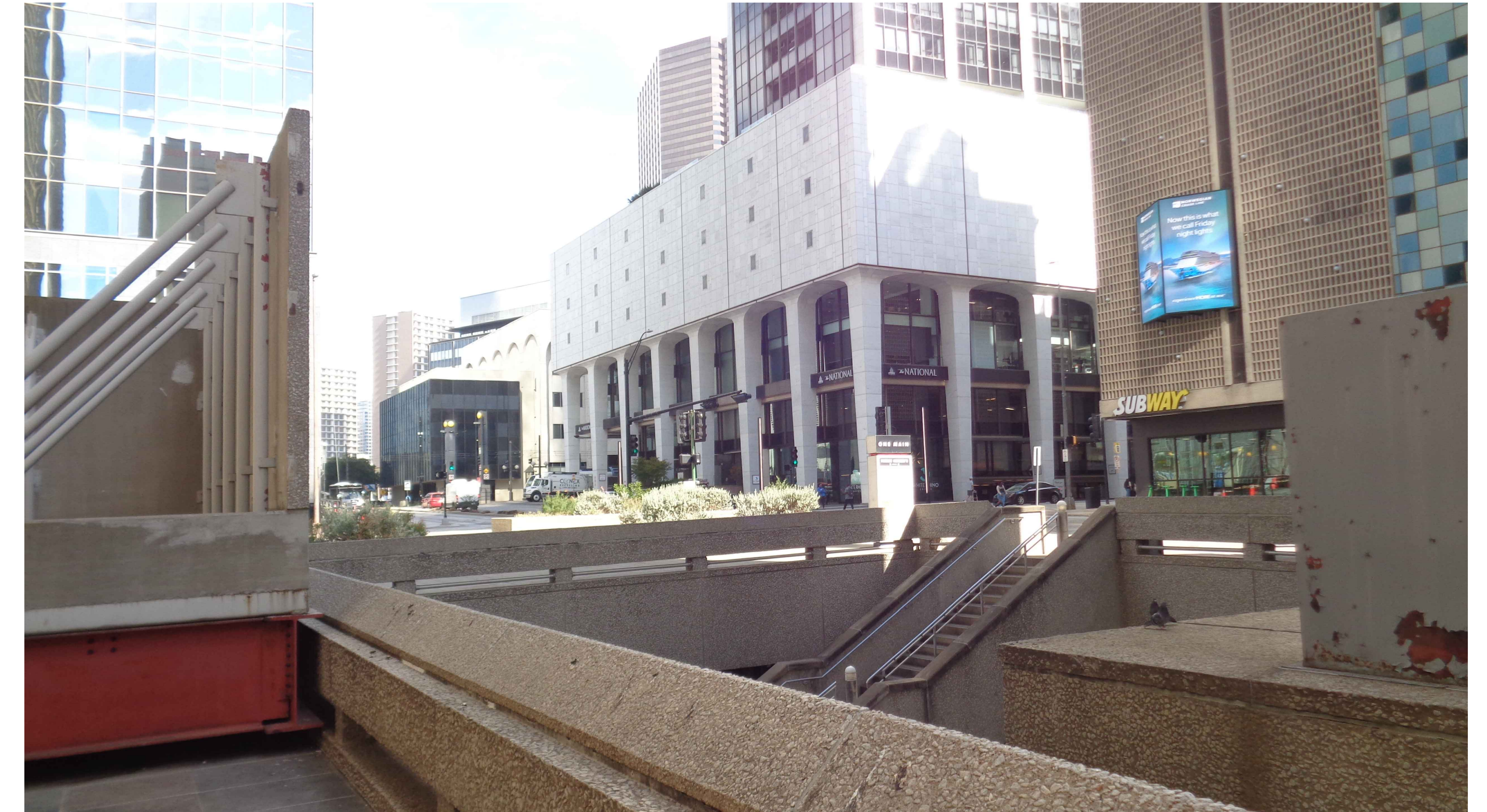
VIEW C - LOOKING NORTHEAST
