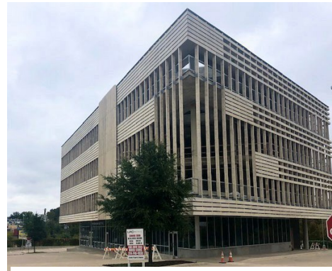
Construction of BookMark Center retail and office space as part of Half Price Books' multi-phased development is nearly complete and available for lease.
