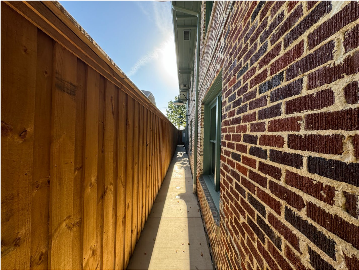
Image 5 - Partial view of north elevation and sloping sidewalk, facing east.
