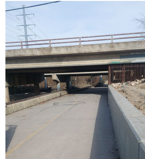
Cottonwood Trail at Forest Lane Overpass
