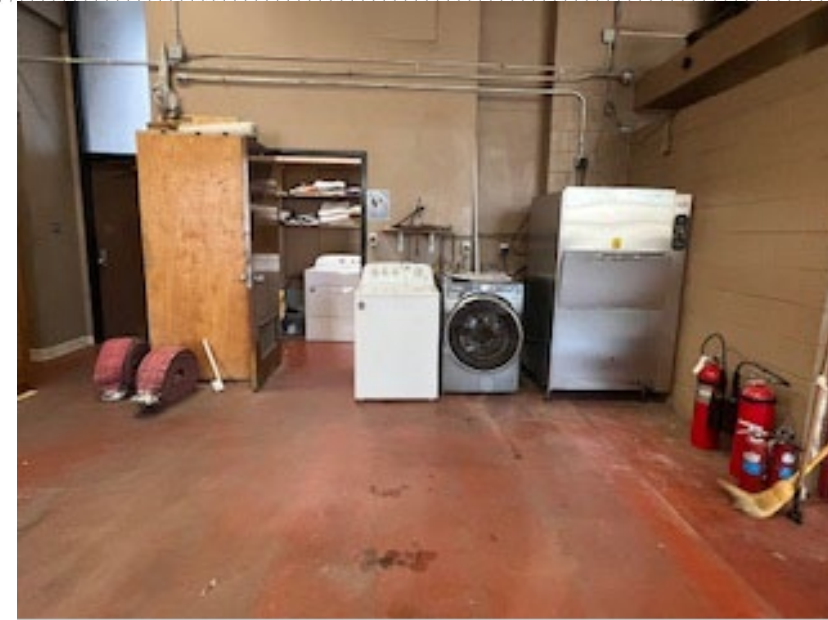
Laundry area in apparatus bay
