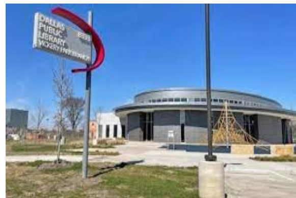
Completed construction & opened New Vickery Park Library
