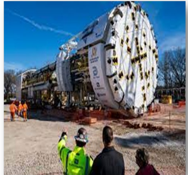
"Big Tex", AKA the Mill Creek Project tunneling equipment
