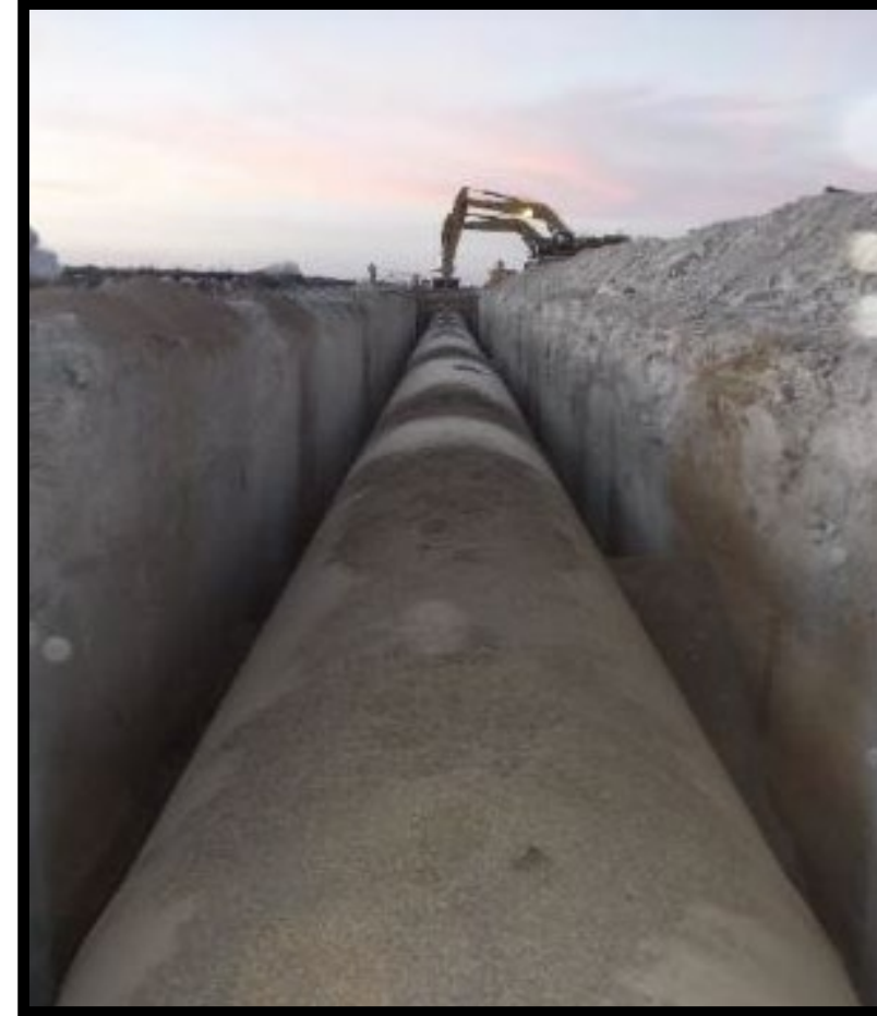
Installation of 108-inch pipe along IPL Section 17
