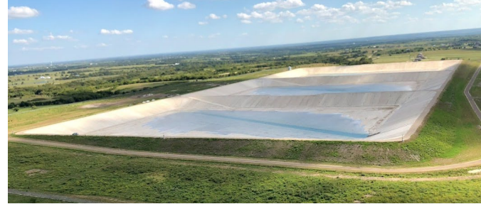
Midlothian Balancing Reservoir
