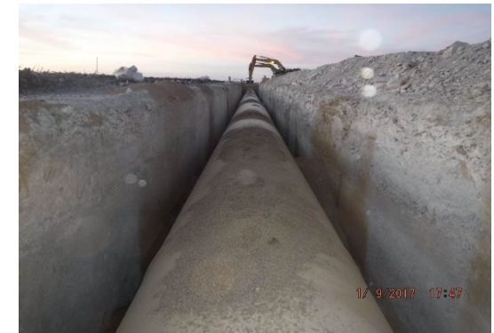
Installation of 108-inch pipe along Section 17
