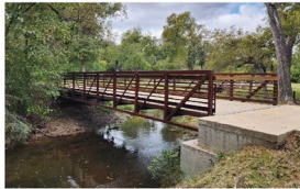
Steel Pedestrian Bridge
