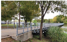
Steel Pedestrian Bridge
