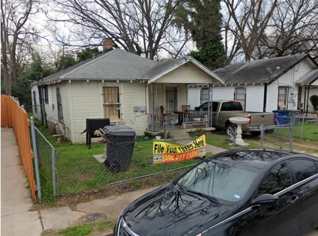
Left, northwest elevation. Source: Google Maps Streetview. February 2020.
