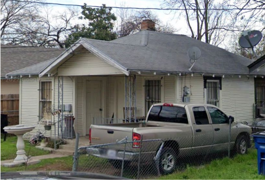
Right, southeast elevation. Source: Google Maps Streetview. February 2020.
