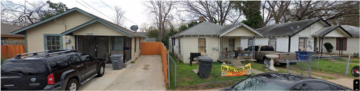
Same blockface as subject property. Source: Google Maps – Street View. February 2020.
