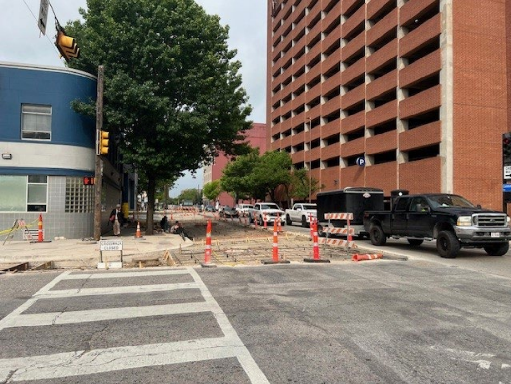
East façade- View from Lamar St.
