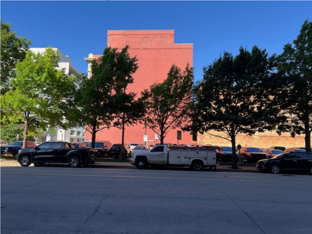
East façade - View from S. Austin St.
