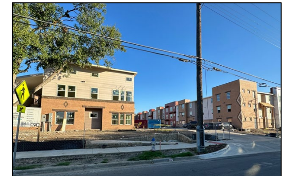
Kiva East construction is almost complete 10/2/2023
