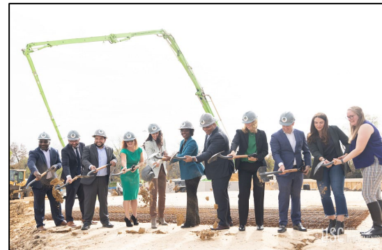
Breaking Ground at Kiva East 12/6/2022
