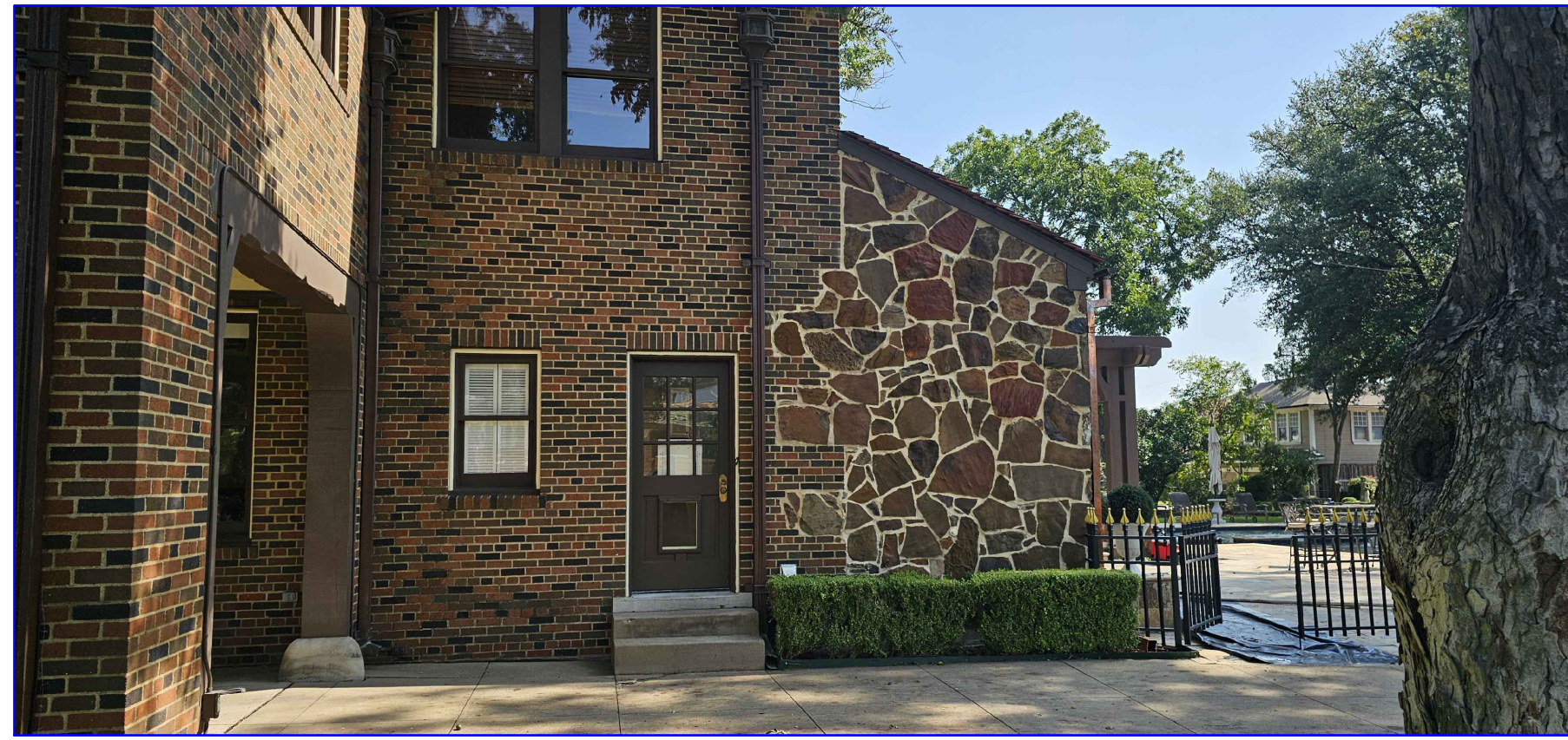
EXISTING SIDE ELEVATION DOOR TO BE REPLACED
